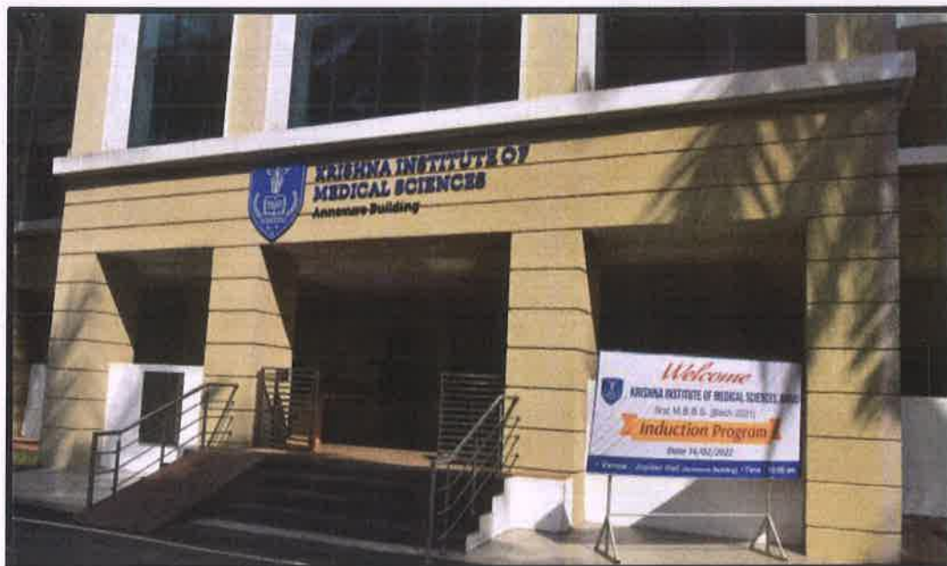
Induction program Venue- KIMS annexure building
